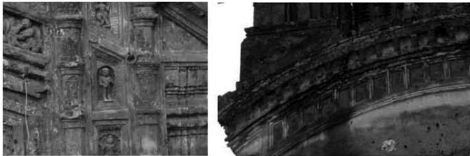
Loss of glazed surface, salt efflorescence, biological growth in terracotta plaques in Damodar Temple, Duttapara, Joypur, Bankura, Source-Author
