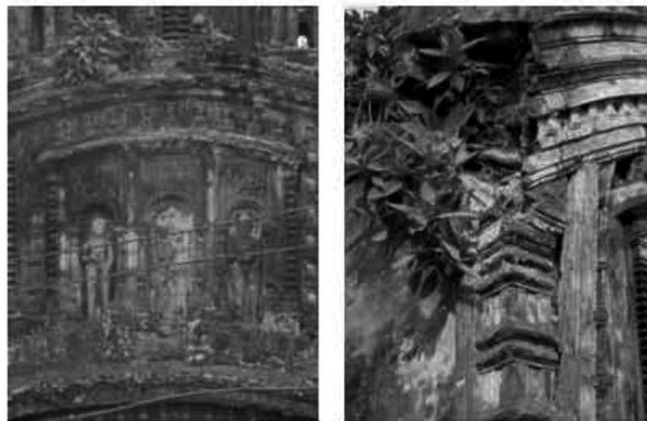
Surface soiling in terracotta plaques in Damodar Temple, Duttapara, Joypur, Bankura and Biological growth in Routkhanda Temple, Joypur, Bankura. Source - Author
